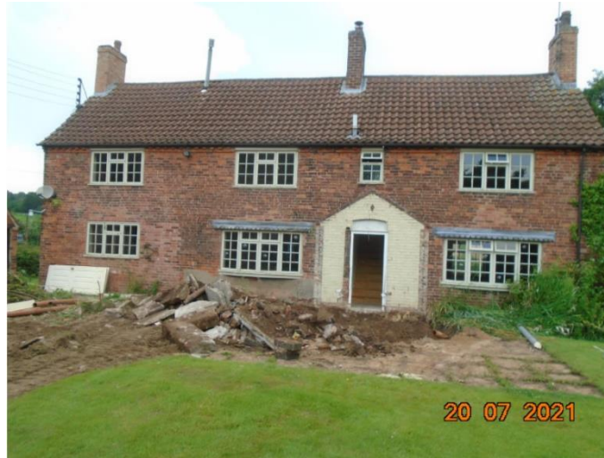
Rear Elevation of farmhouse prior to unauthorised works being undertaken
